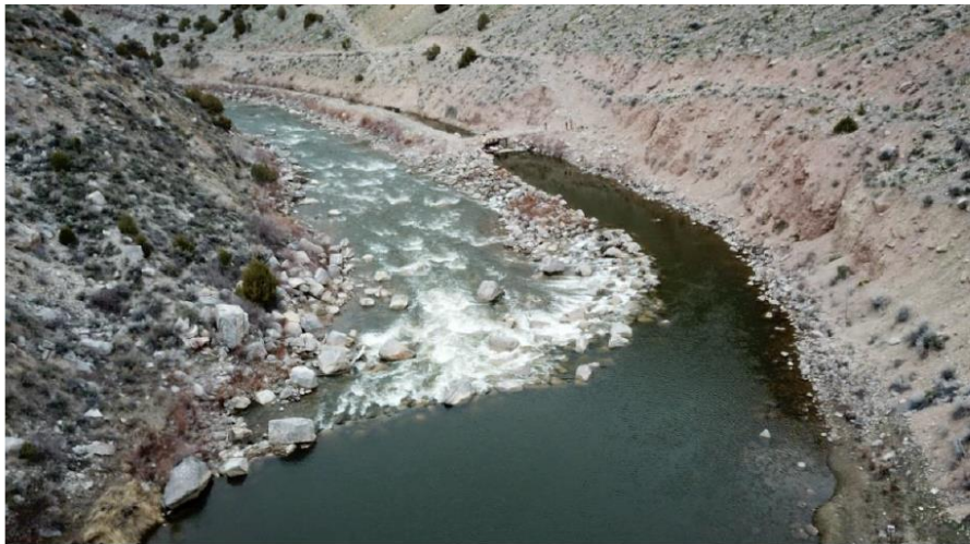
Figure 2. Existing conditions at low water (553 cfs) show the diversion of water into the Maybell Ditch to the right and the steep drop-off toward the main channel of the Yampa to the left. (Photo: J-U-B Engineers)
